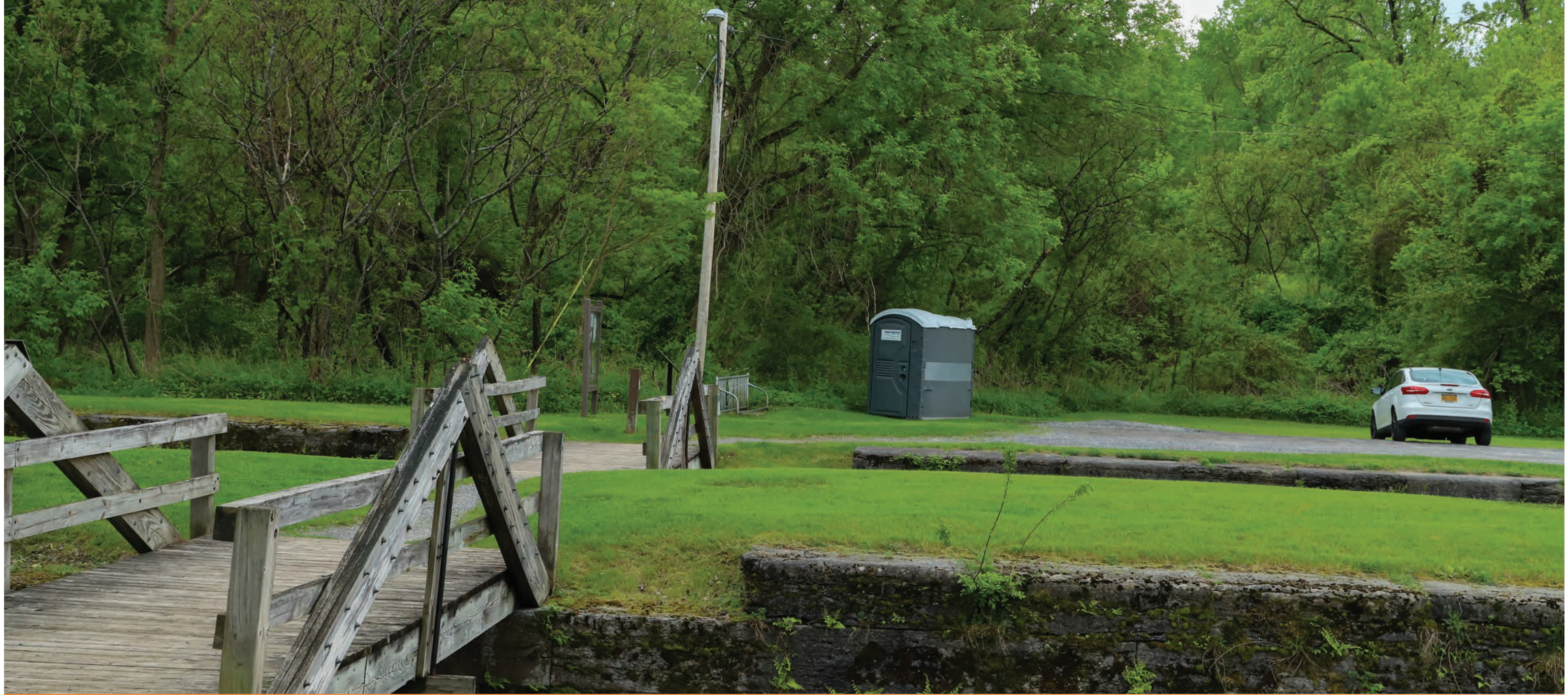
VP 3 - Schoharie Crossing - Yankee Hill Lock EXISTING CONDITION
