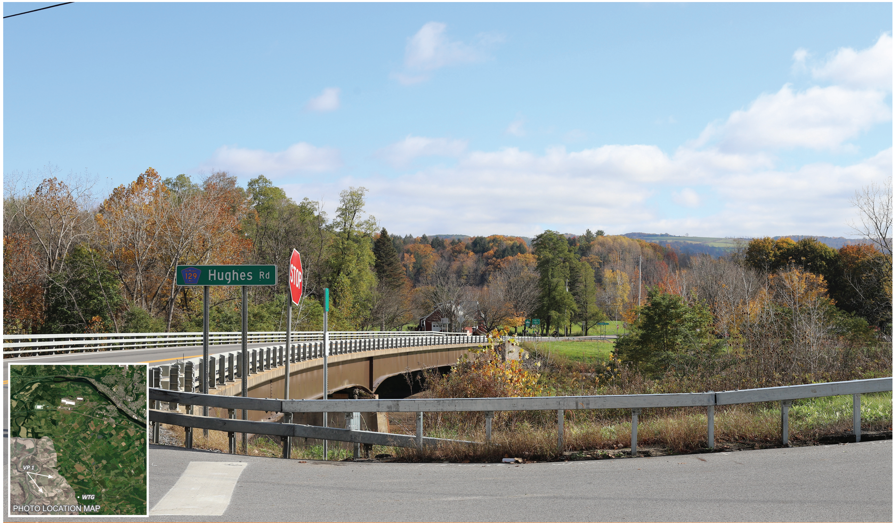
VP 1 EXISTING CONDITION
