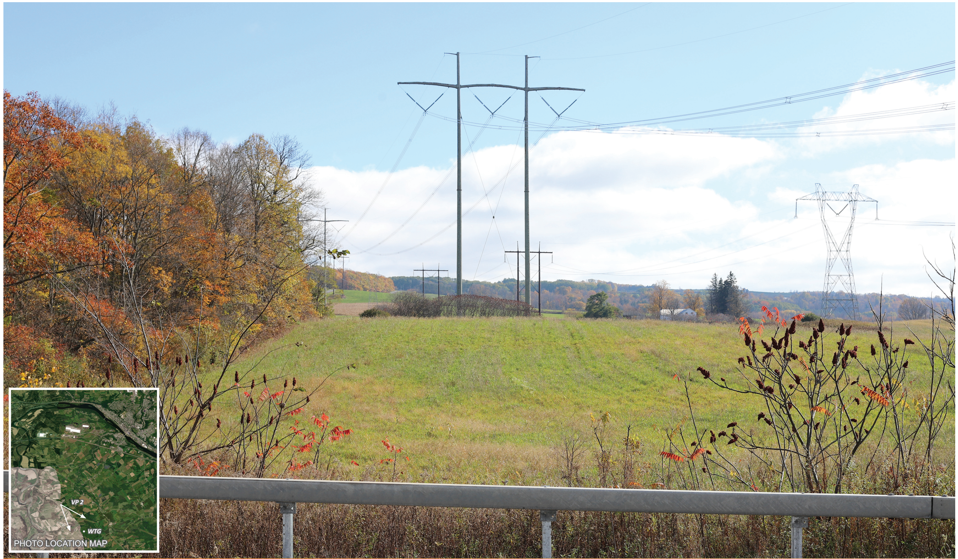
VP 2 EXISTING CONDITION
