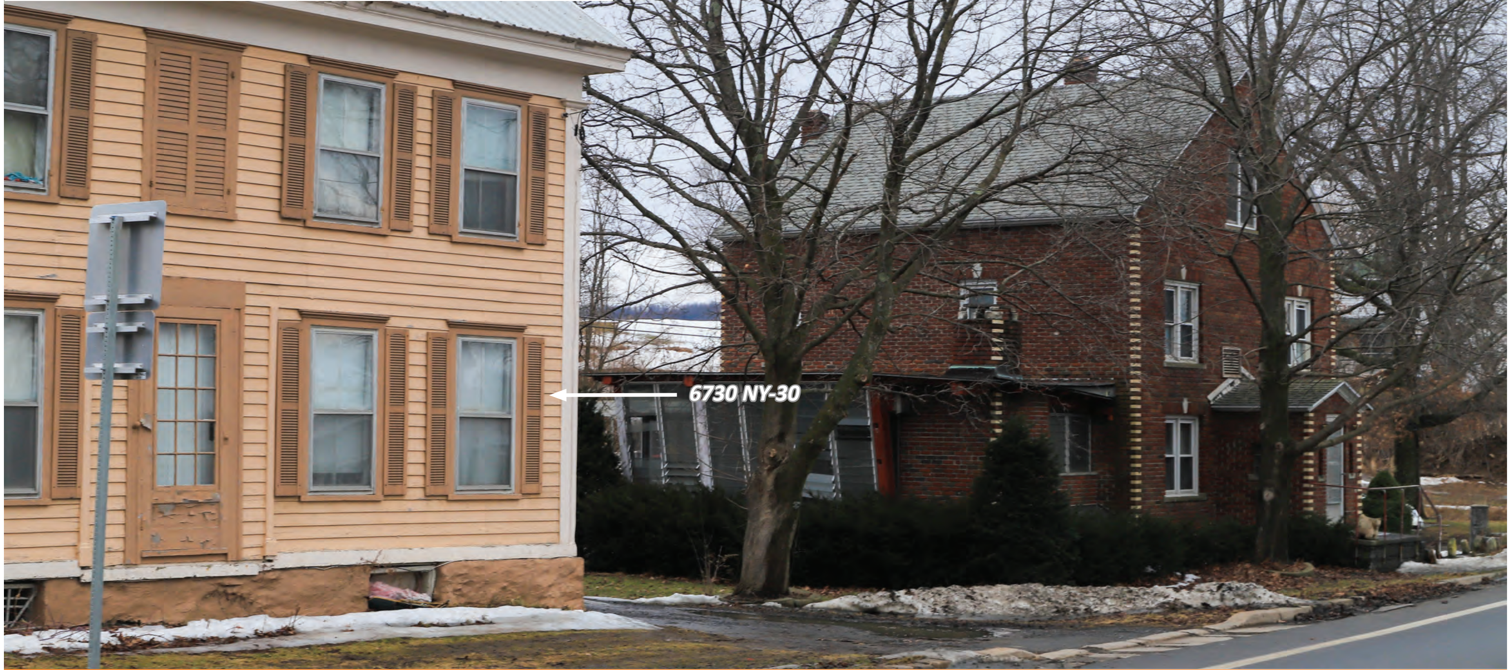
VP 3 - 6714 NY-30 EXISTING CONDITION
