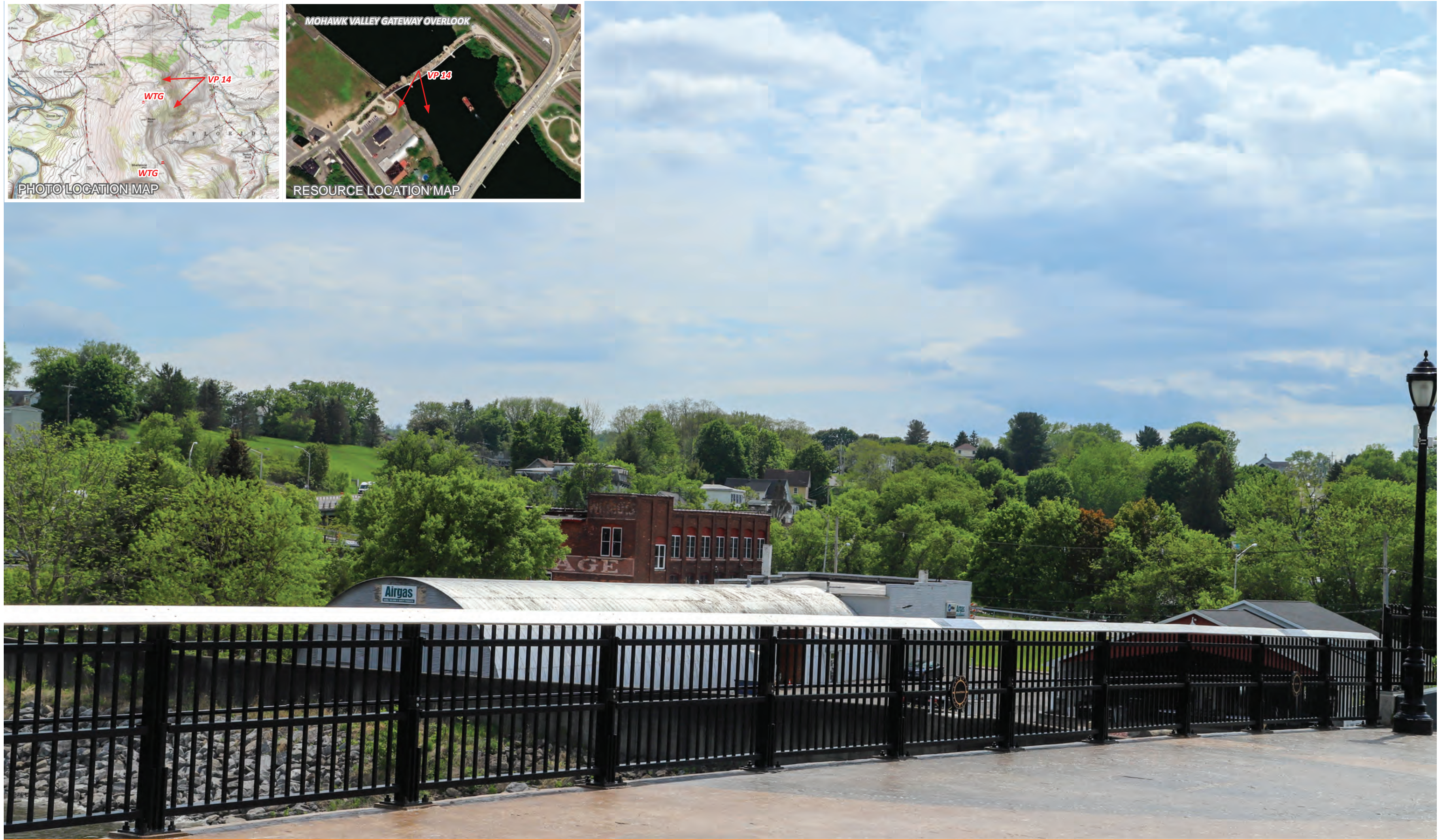
VP 14 - Mohawk Valley Gateway Overlook EXISTING CONDITION
