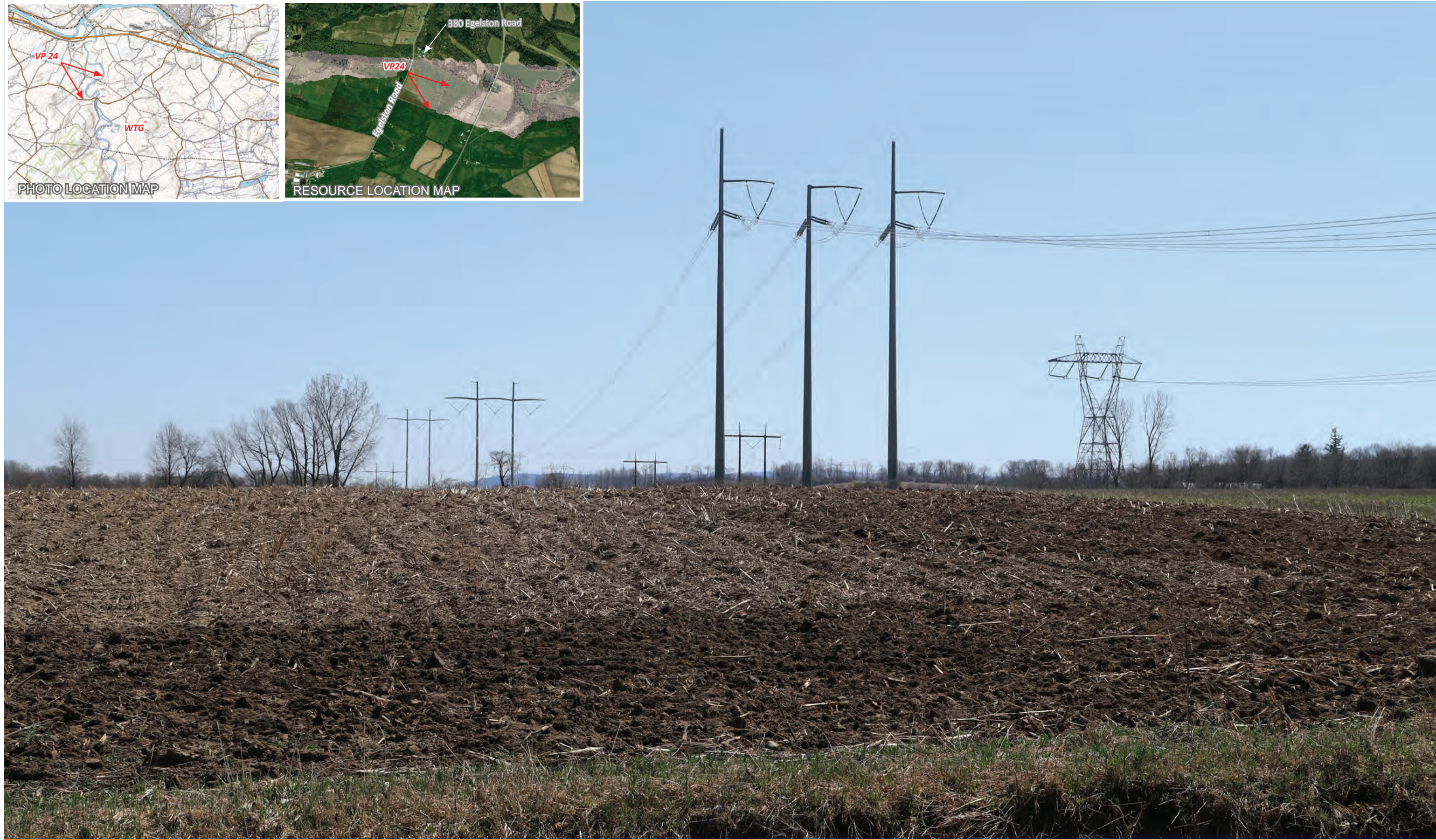
VP 24 - Egelston Road EXISTING CONDITION
