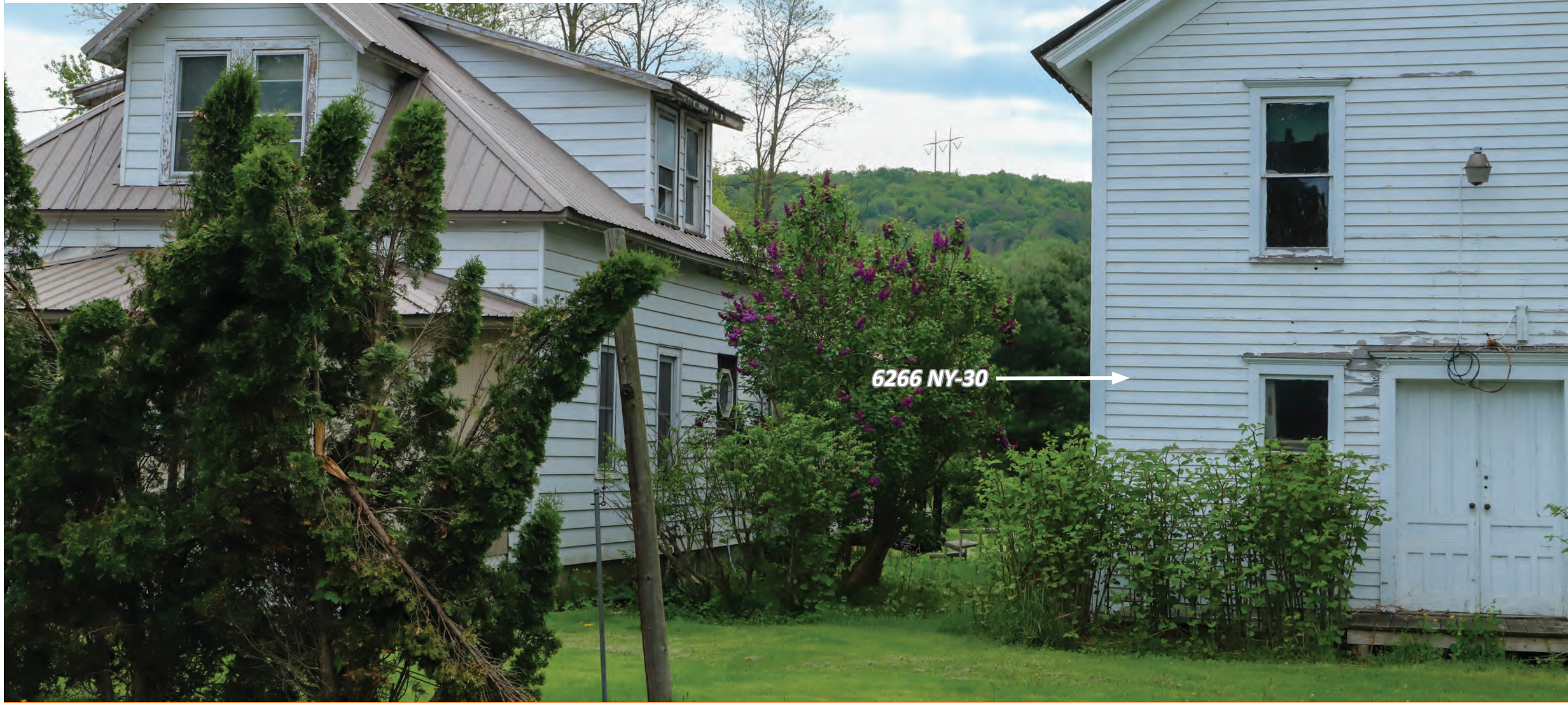
VP 5 - 6266 NY-30 EXISTING CONDITION
