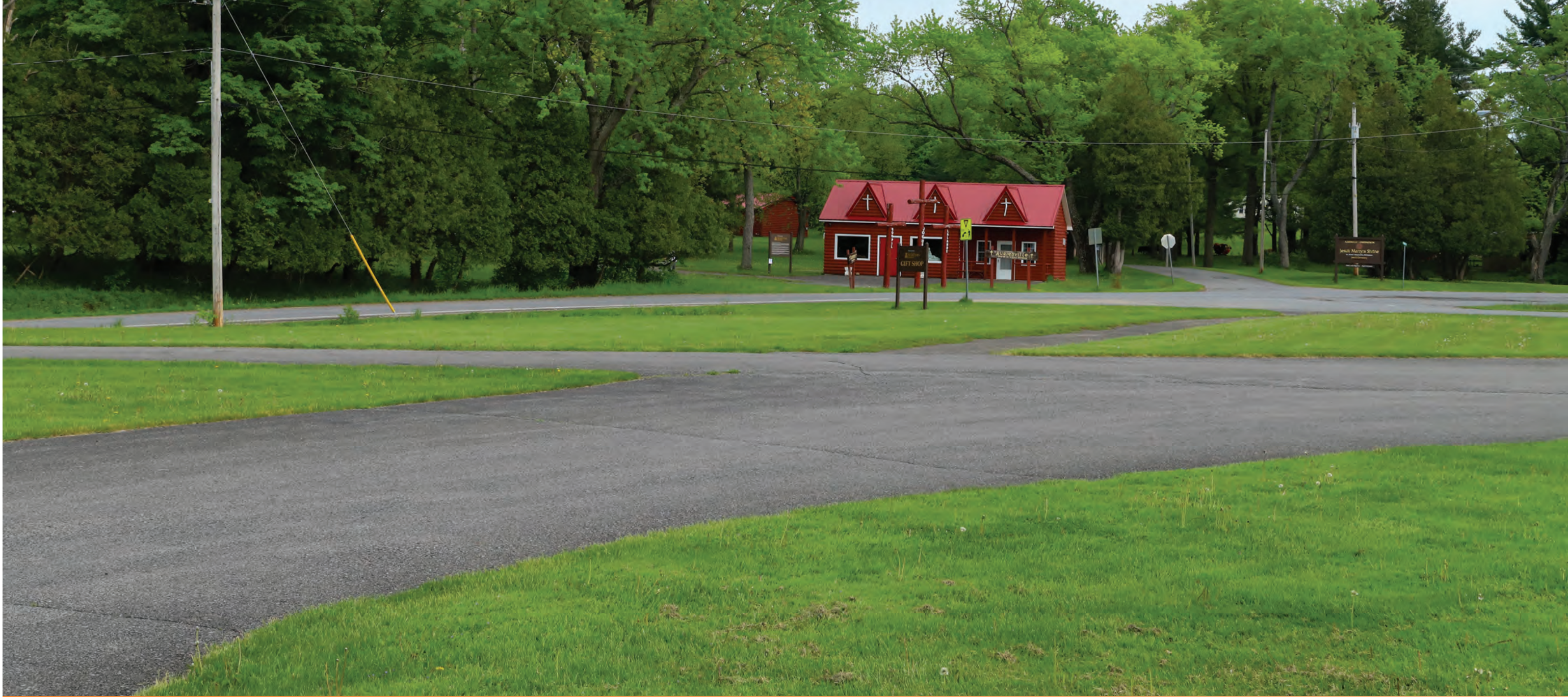
VP 11 - Auriesville Shrine - Martyrs Shrine Visitor Center EXISTING CONDITION
